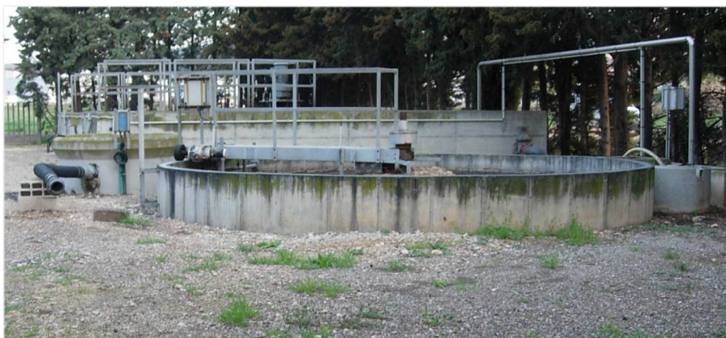
Ancienne Station d'Epuration
