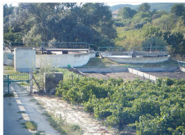
Ancienne Station d'Epuration
